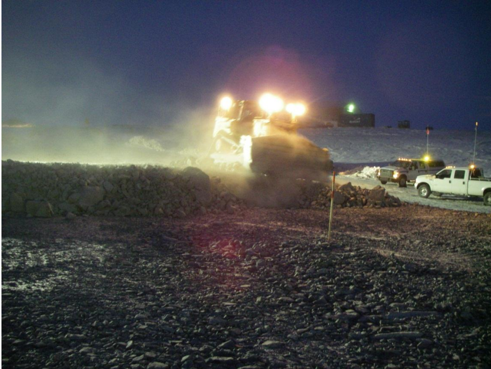
Photo 7: North Dam – CAT D8 dozer placing ROQ on the final lift of the dam shell. Photo looking north-east from station 1+00.
