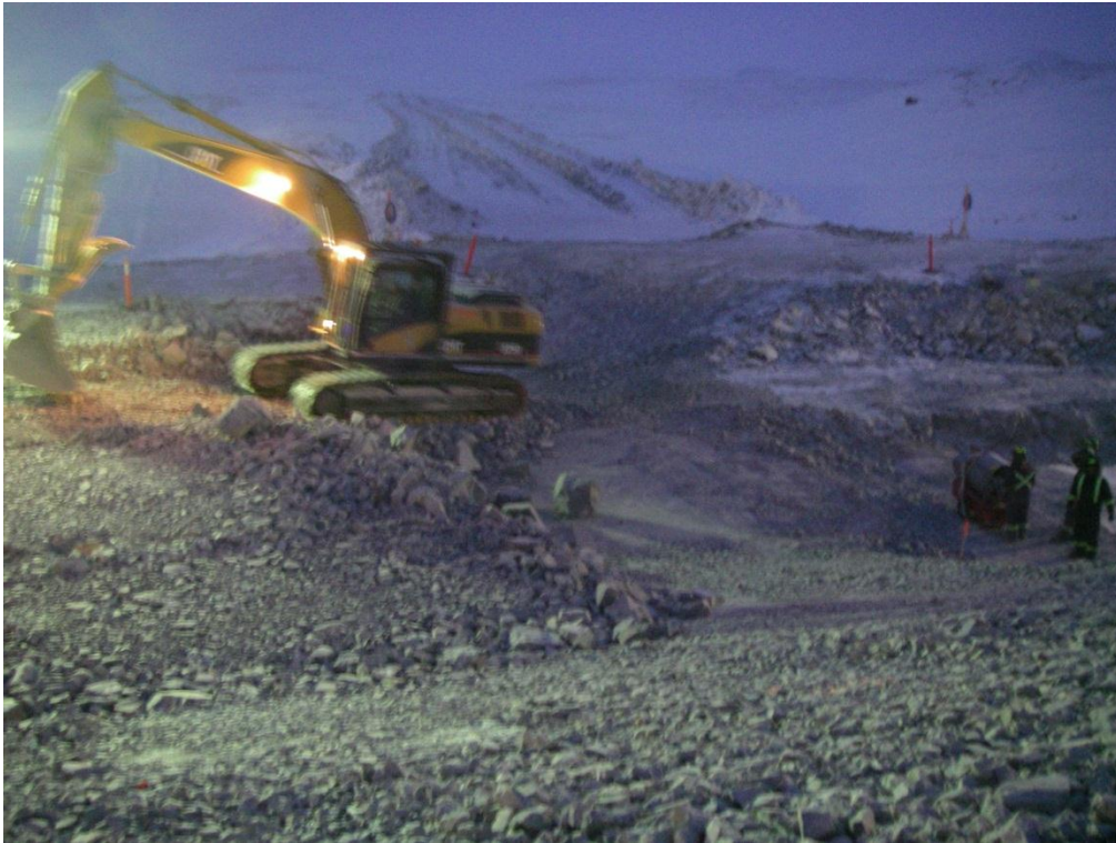
Photo 5: North Dam – excavator shaping the first lift of ROQ to create vehicle access ramp into the key trench. Photo looking east around station 0+90
