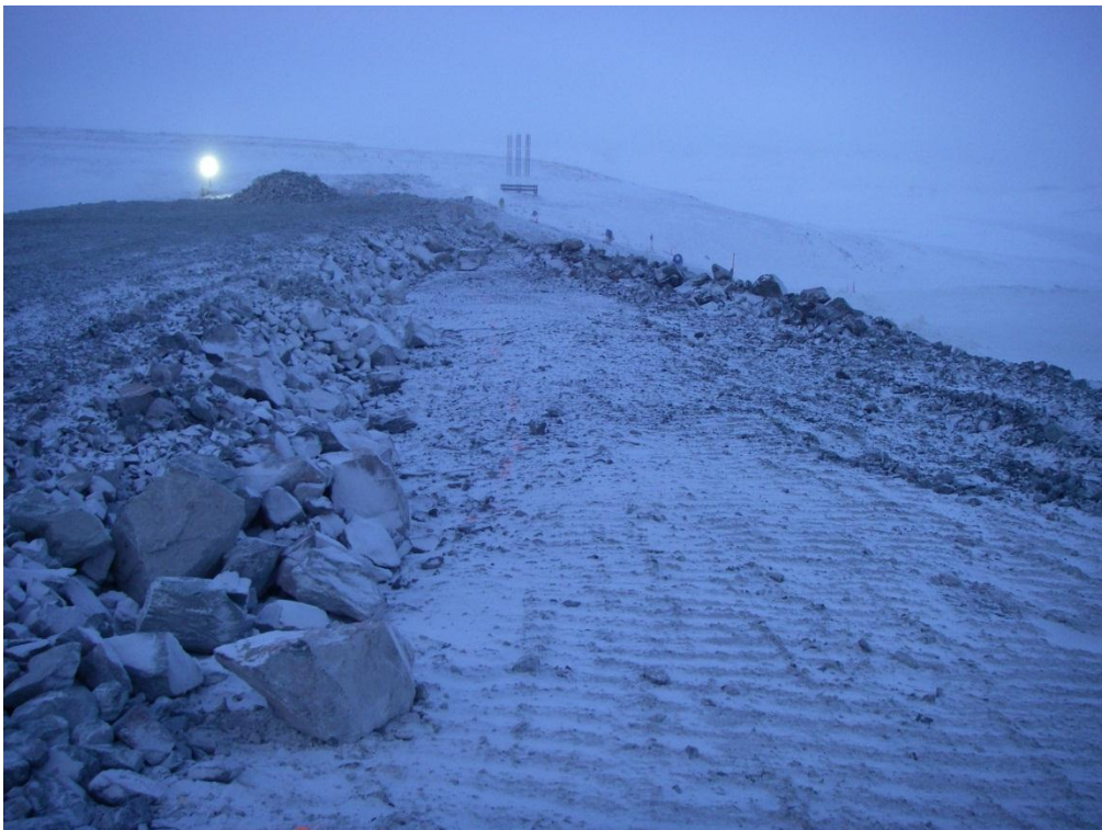
Photo 10: Excavator placing ROQ material on diversion berm. Photo North Dam – progress photo of the final lift of ROQ. Photo looking south-west along the downstream crest of the dam shell from Sta. 1+90.
