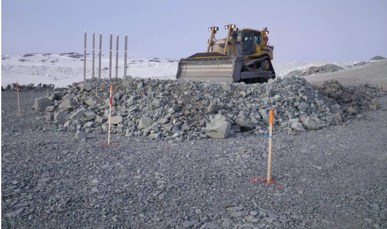
Photo 3: North Dam - CAT D8 dozer starting to place final/upper lift of ROQ on the North dam.
