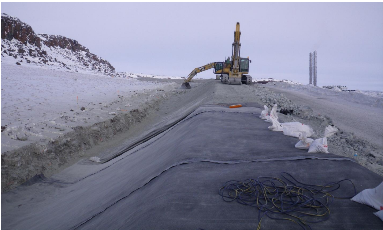
Photo 4: Diversion Berm - Excavator placing ROQ material on diversion berm. Photo looking east along diversion berm.
