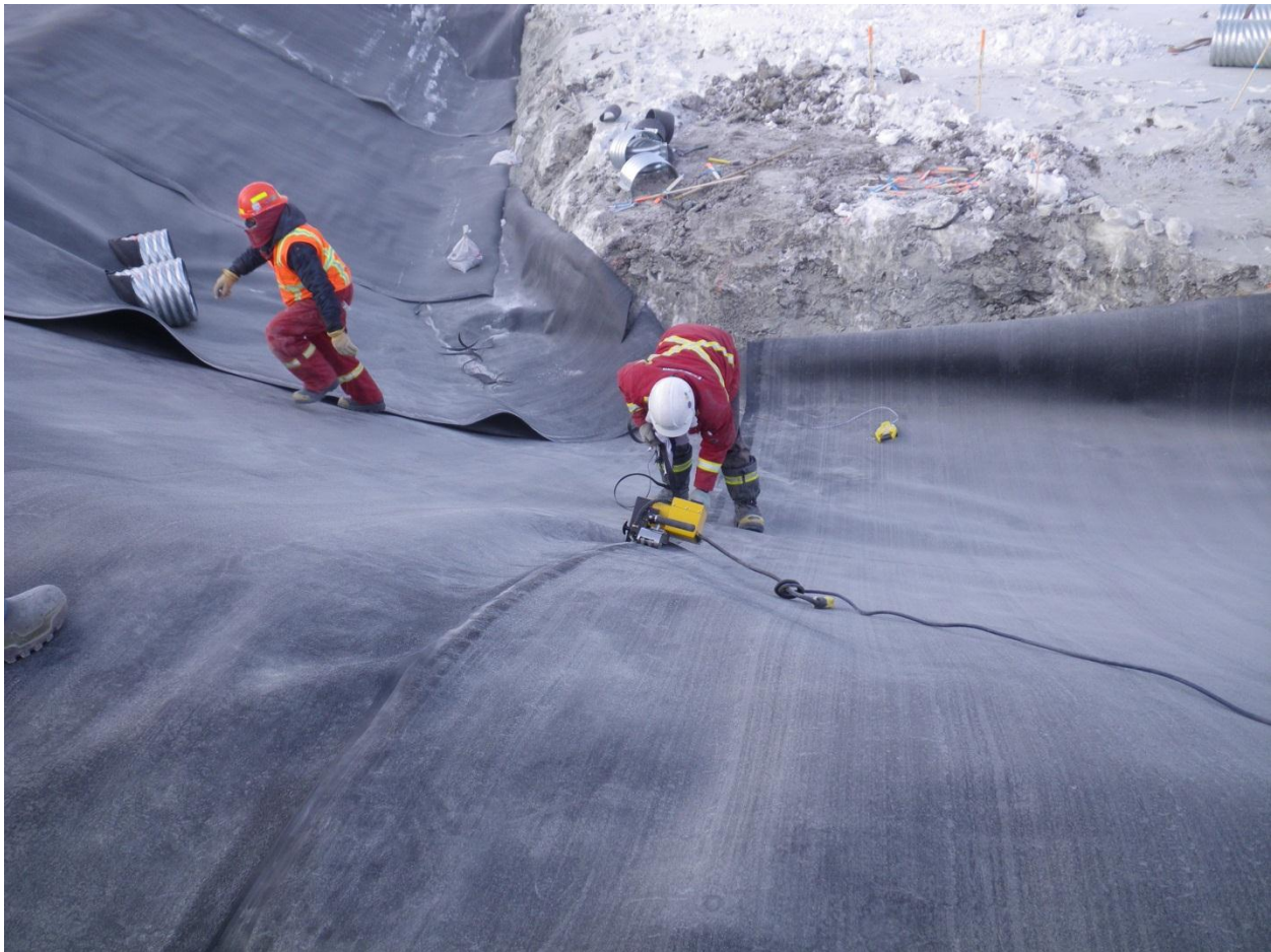
Photo 2: Diversion Berm - Layfield seaming HDPE liner near station 020 of the diversion berm.
