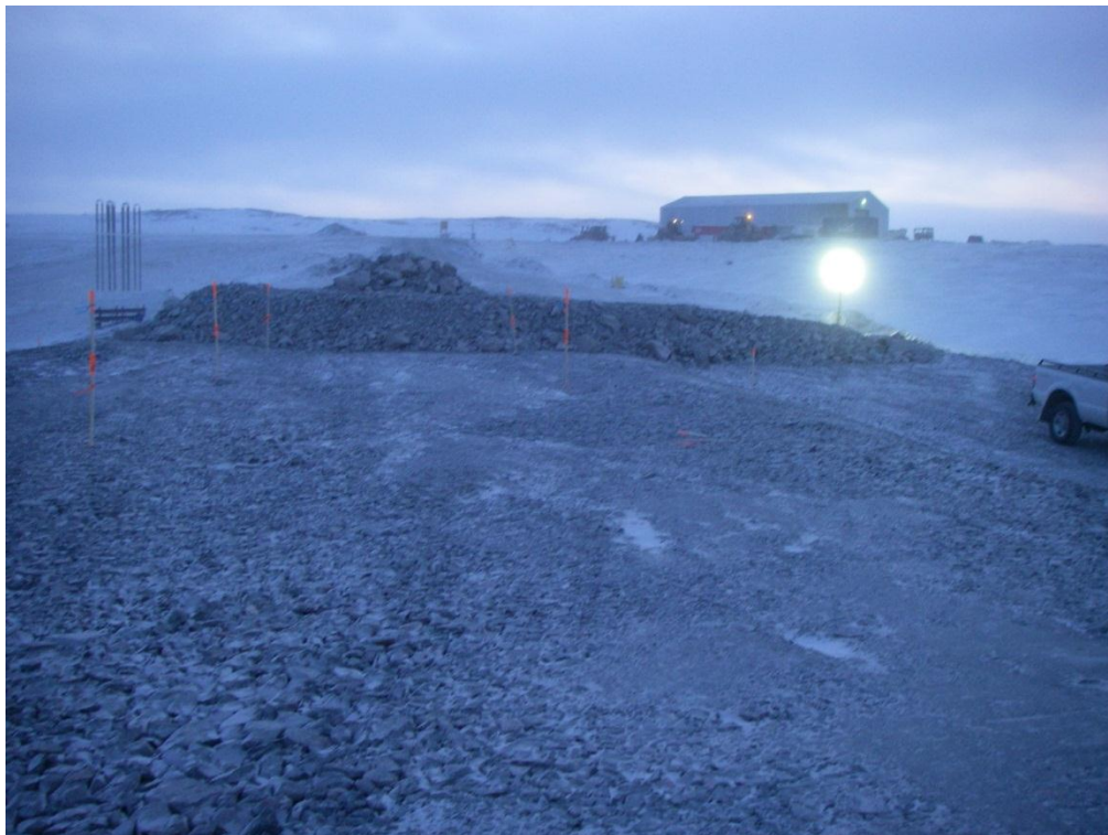
Photo 7: North Dam – CAT D8 dozer placing ROQ on the final lift of the dam shell. Photo looking north-east from station 1+00.
