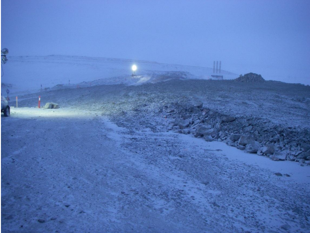
Photo 9: North Dam – progress photo of the final lift of ROQ. Photo looking south-west along the upstream crest of the dam shell from Sta. 1+90.
